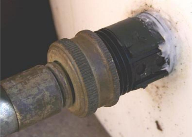
The connection between barrels is made with a washing machine hose (yet another leftover, about \$6 if you buy new) because it has the needed female hose fittings on each end. You can add inline shutoff valves to allow isolating each barrel (great if the hose springs a leak).
