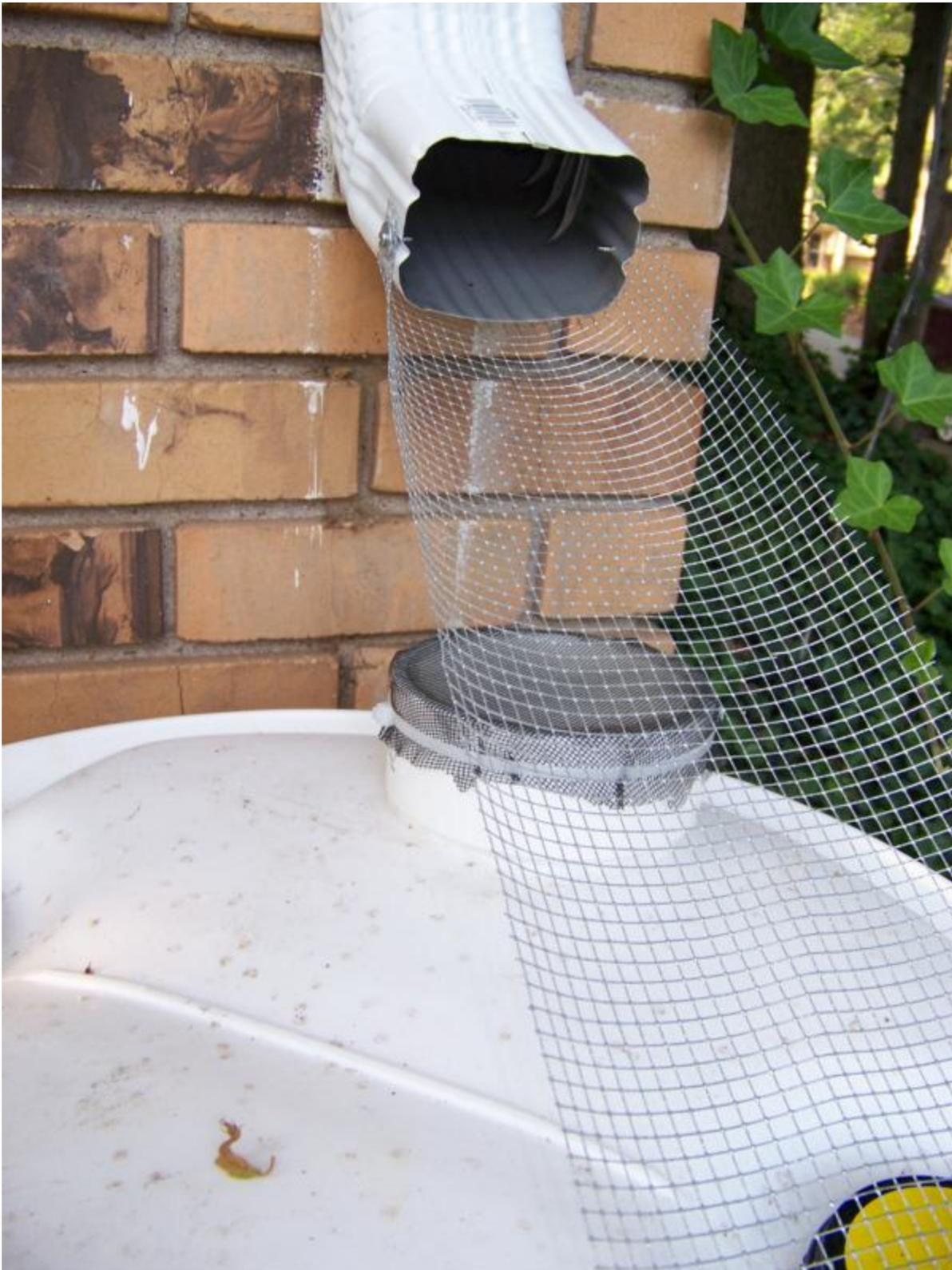
**The house has overhanging trees, so the intake screens consist of hardware cloth at an angle (so the leaves will be washed away and to keep them off the mosquito screen) plus the mosquito screen over the funnel.**
