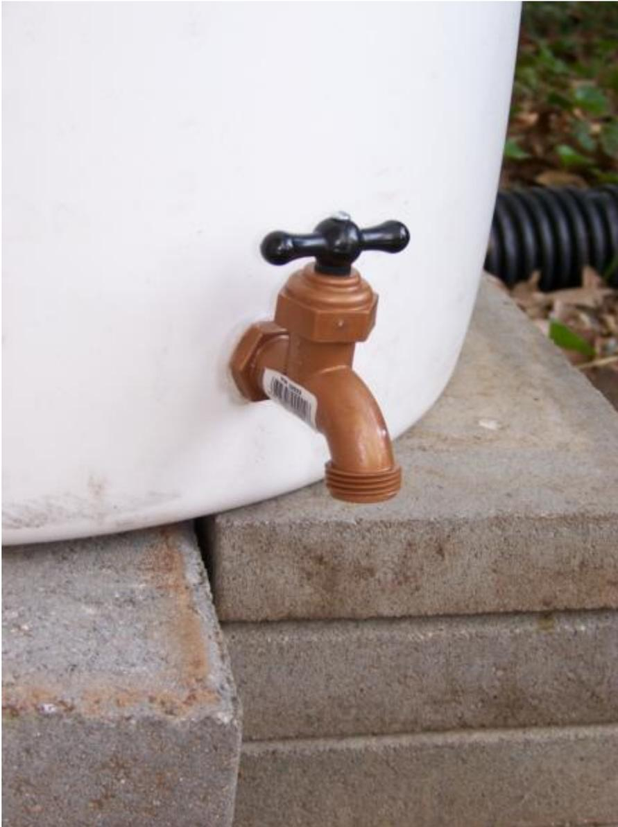
**The base is made of six 12" x 12" pavers and three 6" x 18" pavers which raise the barrel high enough to allow connecting a hose. The hose bibb is**
