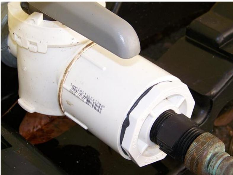
A two inch threaded to 2 inch PVC pipe adapter screws on the valve, then a 2 inch slip to 3/4 inch threaded pipe adapter is glued in to provide a place to screw in a 3/4 inch pipe to male hose thread adapter.
