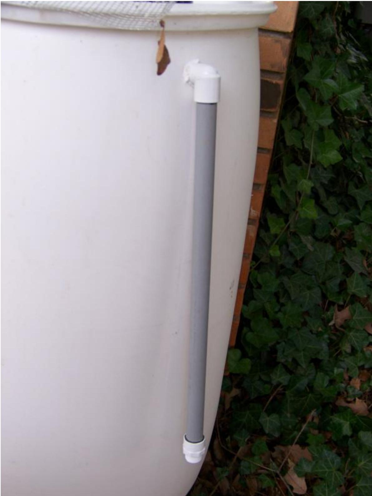
**The overflow pipe and hose bibb are carefully threaded into just-the-right-size holes drilled and filed in the barrel and are sealed with caulk.**
